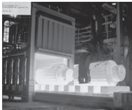
Steel forging furnace
