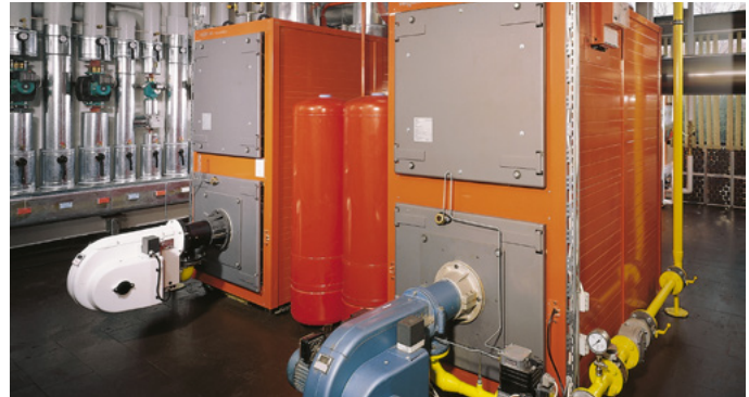
Gas inlet pressure monitoring on high-performance boilers
